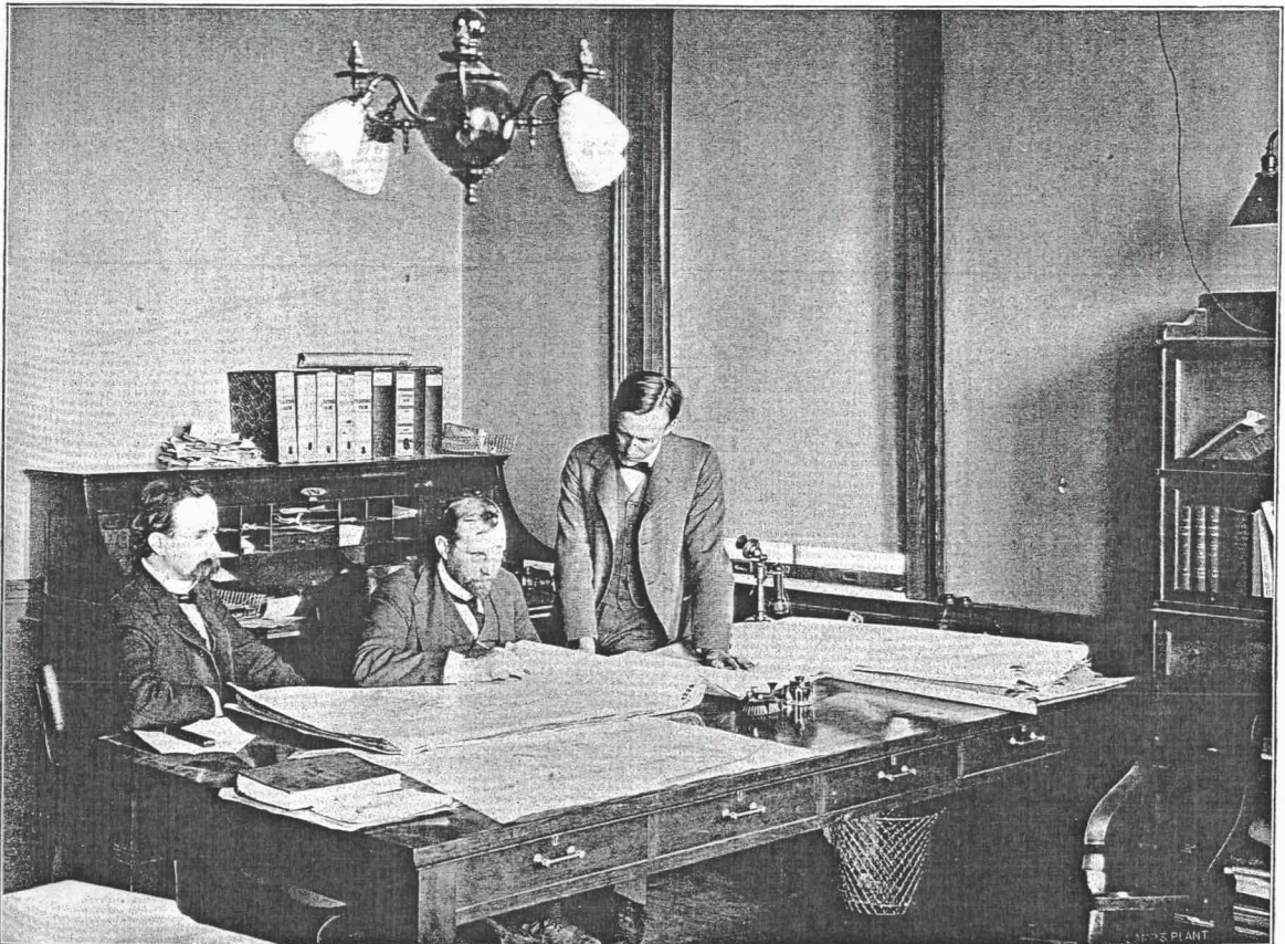
Office of Chief Engineer, Minnequa Works, Pueblo.
